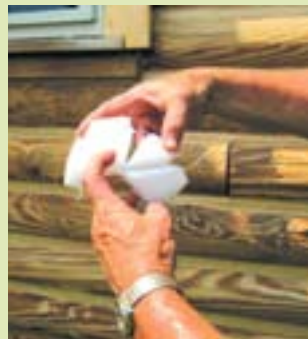
Cut triangular blocks of EPS or polyethylene foam
