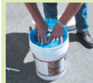
Replace plastic liner over the surface of the sealant
