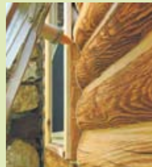
Fill the 3/8" gap between the surface of the foam and the edge of the frame with sealant
