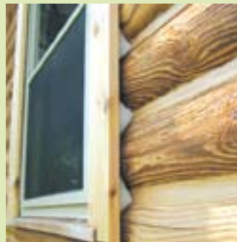
Insert foam blocks into void between logs and frame. Leave 3/8" gap between surface of foam and edge of frame
