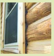
Insert Log Gap Cap<sup>™</sup> into void between logs and frame. Leave 3/8" gap between surface of foam and edge of frame
