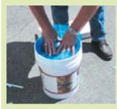
Replace plastic liner over the surface of the sealant
