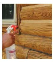
• **Tip:** If you used masking tape at the edges of the *Energy Seal*, remove it now and smooth out edges with your tool.
