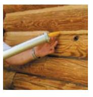
After the joint is filled, trowel out to approximately 3/8th of an inch thick across the entire joint, making sure
